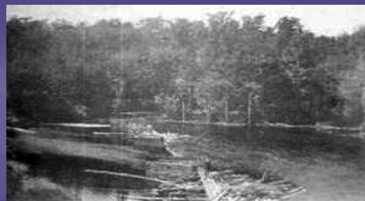
Lumberman's dam c 1890 between mill and bridge to float logs over the rapids on the way to Bracebridge mills. Remnants are still there.
