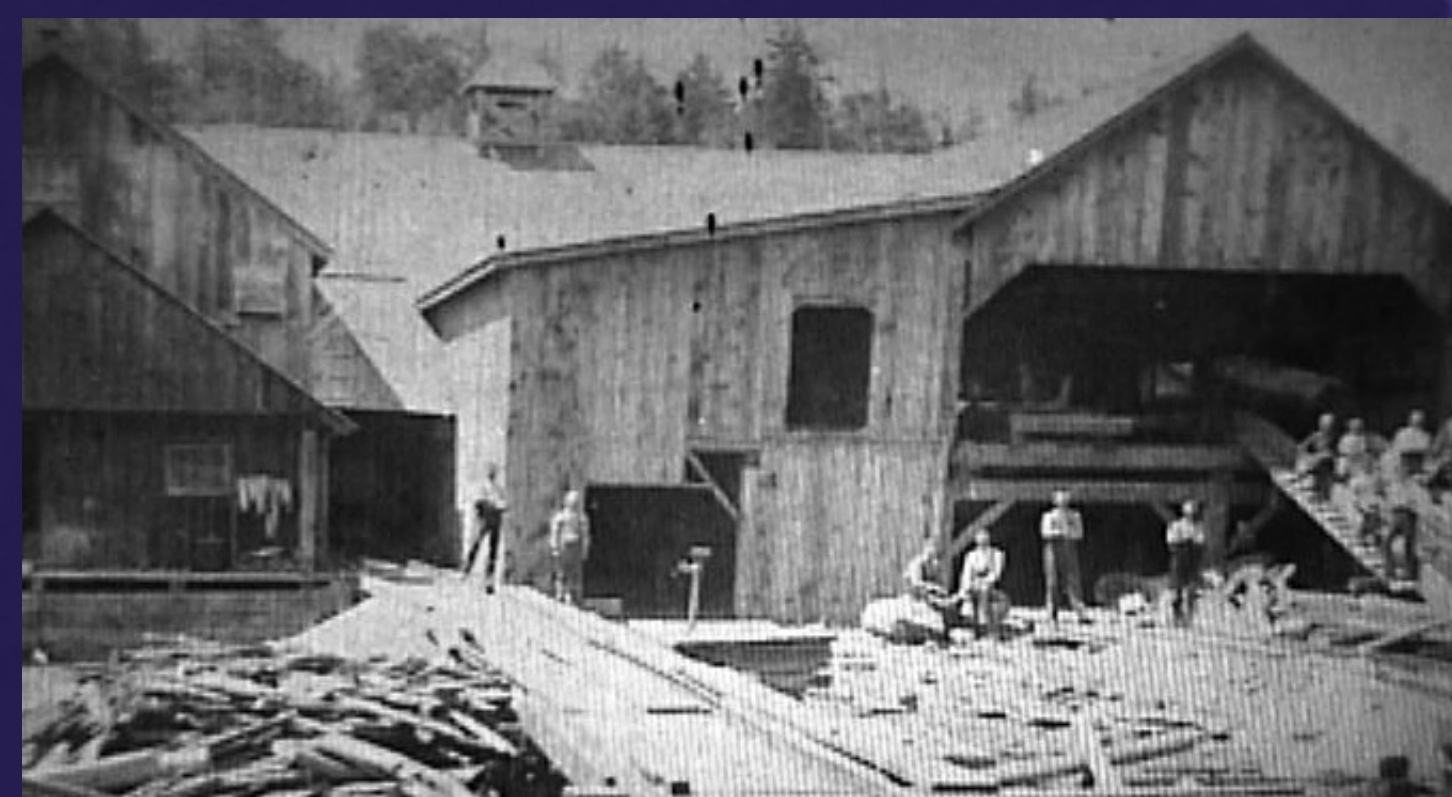
At the sawmill logs were hauled up from the sluiceway by jackladder to the saw.
